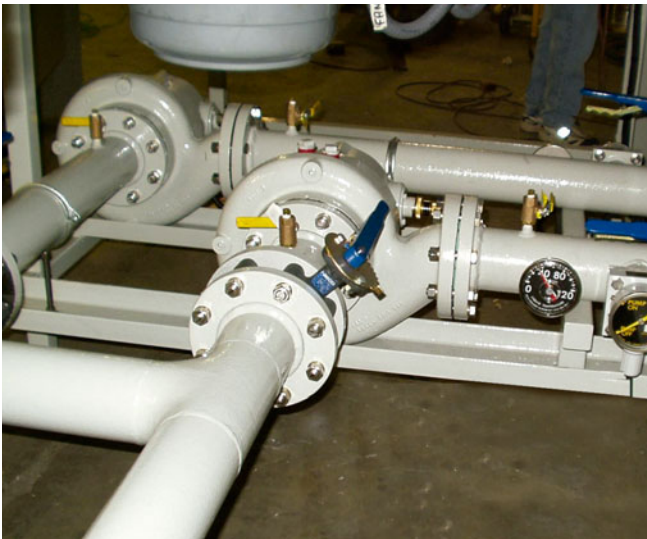
Dual Pump Cooling for Oil-Filled Transformers
