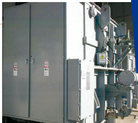
83 KA @ 266 VDC Chlorate 12 Pulse Transformer/Rectifier
