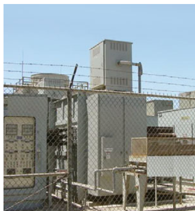
40 KAC @ 200 VDC Power Supply for Zinc Extraction
