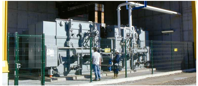
83 KA 12 pulse Transformer/Rectifier Line-up
