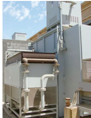
12 MVA Rectifier-Transformer with Oil to Air Cooling
