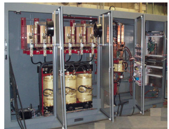
500 ADC @ 1000 VDC High Frequency DC Chopper
