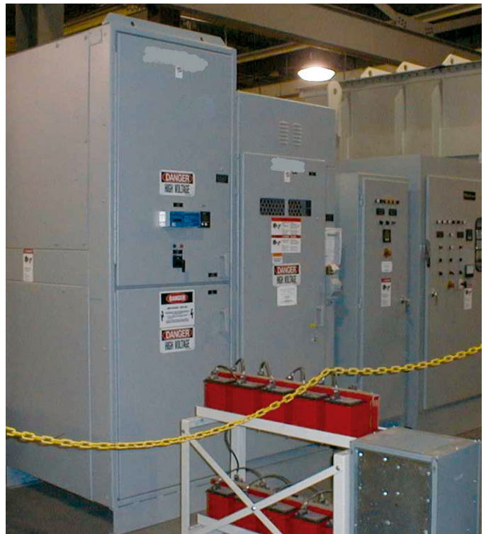
15 KA @ 380 VDC Chlorine Supply
